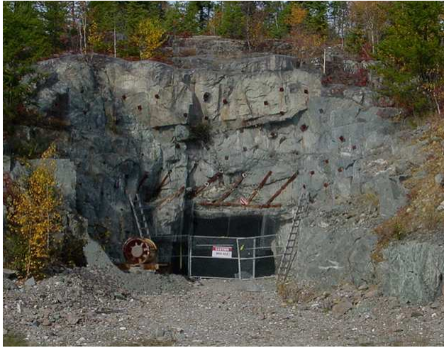
Davidson Tisdale Ramp Portal
