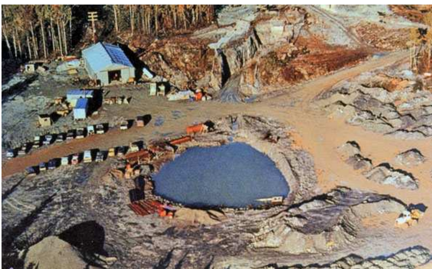
Aerial view of Fuller Mine
